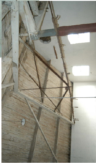
Principal rafters reinforced, additional bracing to trusses
