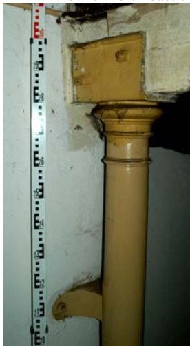
Detail of cast iron stanchion (southern row) - note inserted beam to LHS
