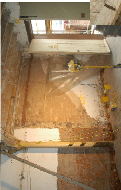
Scarf of gallery wall and blocked original entrance (lighter coloured brick)
