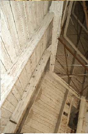
Mortices (probably for glazing bars) in face of uppermost partition
