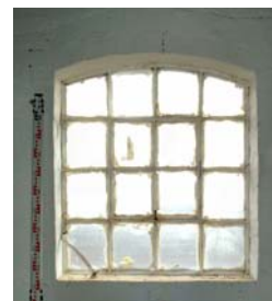
16 pane opening hopper window 1st floor, eastern elevation
