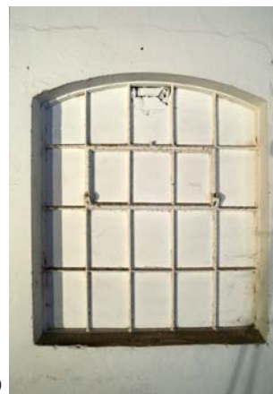
20 pane hopper opening window (northern elevation)
